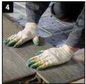
**Install floor finish** Cover the heating cables with self-levelling compound or tile directly on top using a full bed of tile adhesive.
